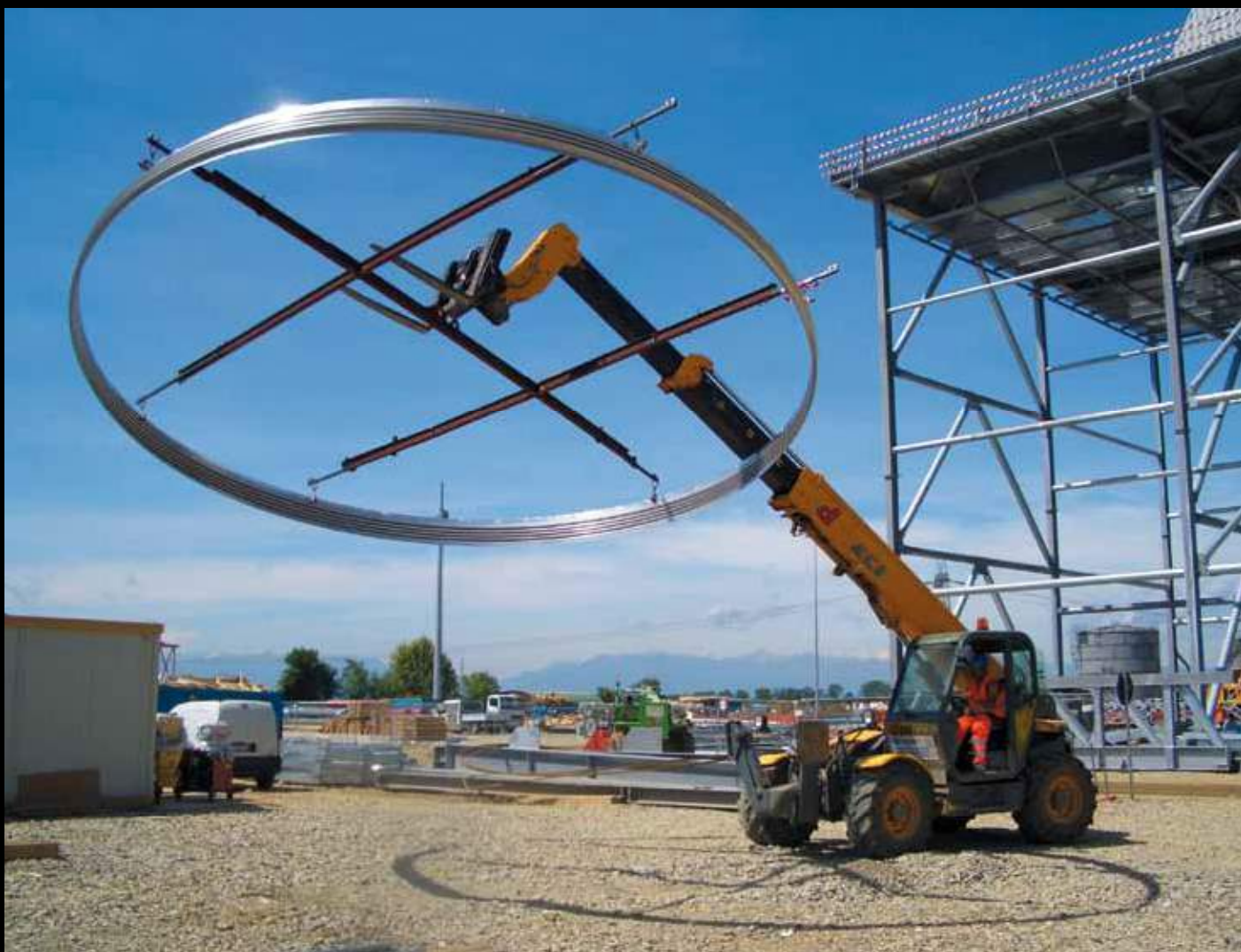
Production of several DN7200 expansion joints directly on a Siemens construction site in Italy
